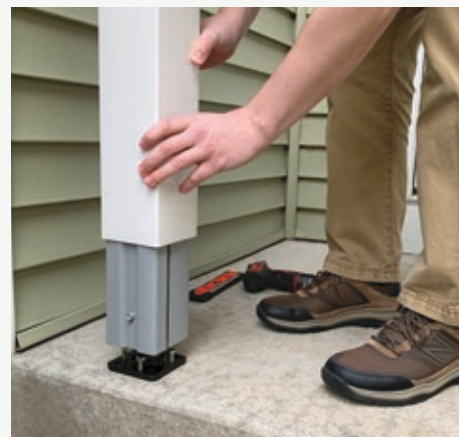
Attach fillers and place sleeve over post.
